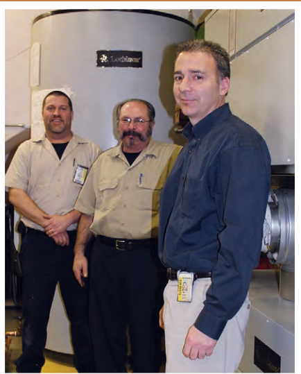
LEFT TO RIGHT , engineers Eric Wright and Rick DiPierri show off Inglis' new energy-efficient boiler with Marc Forte, Director of Facility Engineering.
