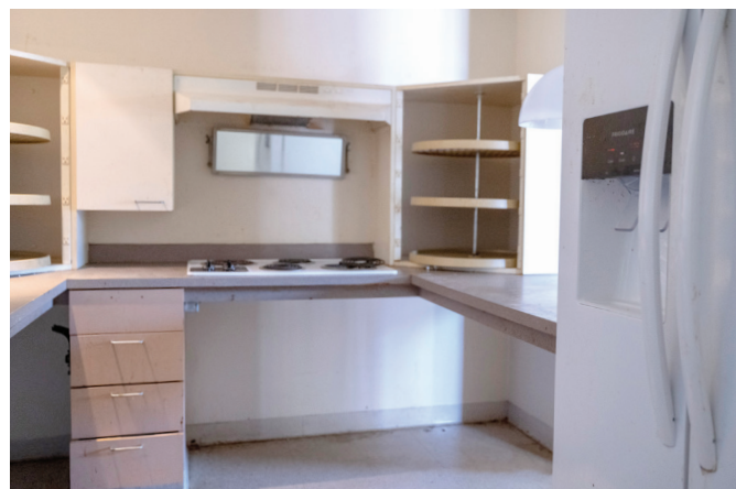
A kitchen, pre-renovation inside Eastwick I.
