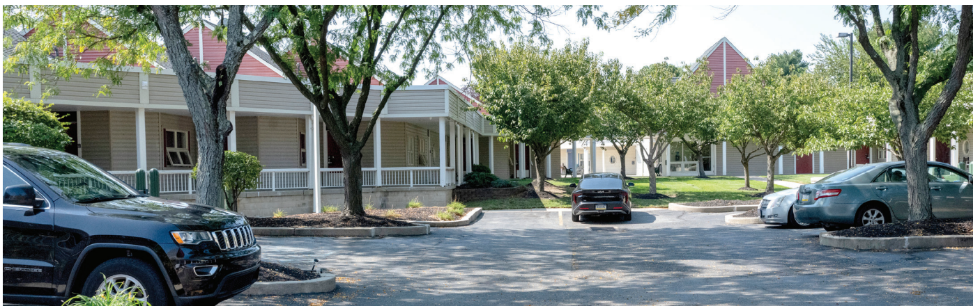
The inner part of the complex of Eastwick I, pre-renovation.
